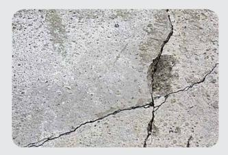
In spite of the best efforts of the architect, engineer and contractor, structures will sometimes move in unanticipated places causing cracks. Resin can be injected into the concrete to accomplish one of two purposes:
